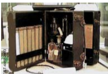
Figure 3: Drunkometer by Hager from the year 1938 (photo: Honolulu Police Department, USA)
